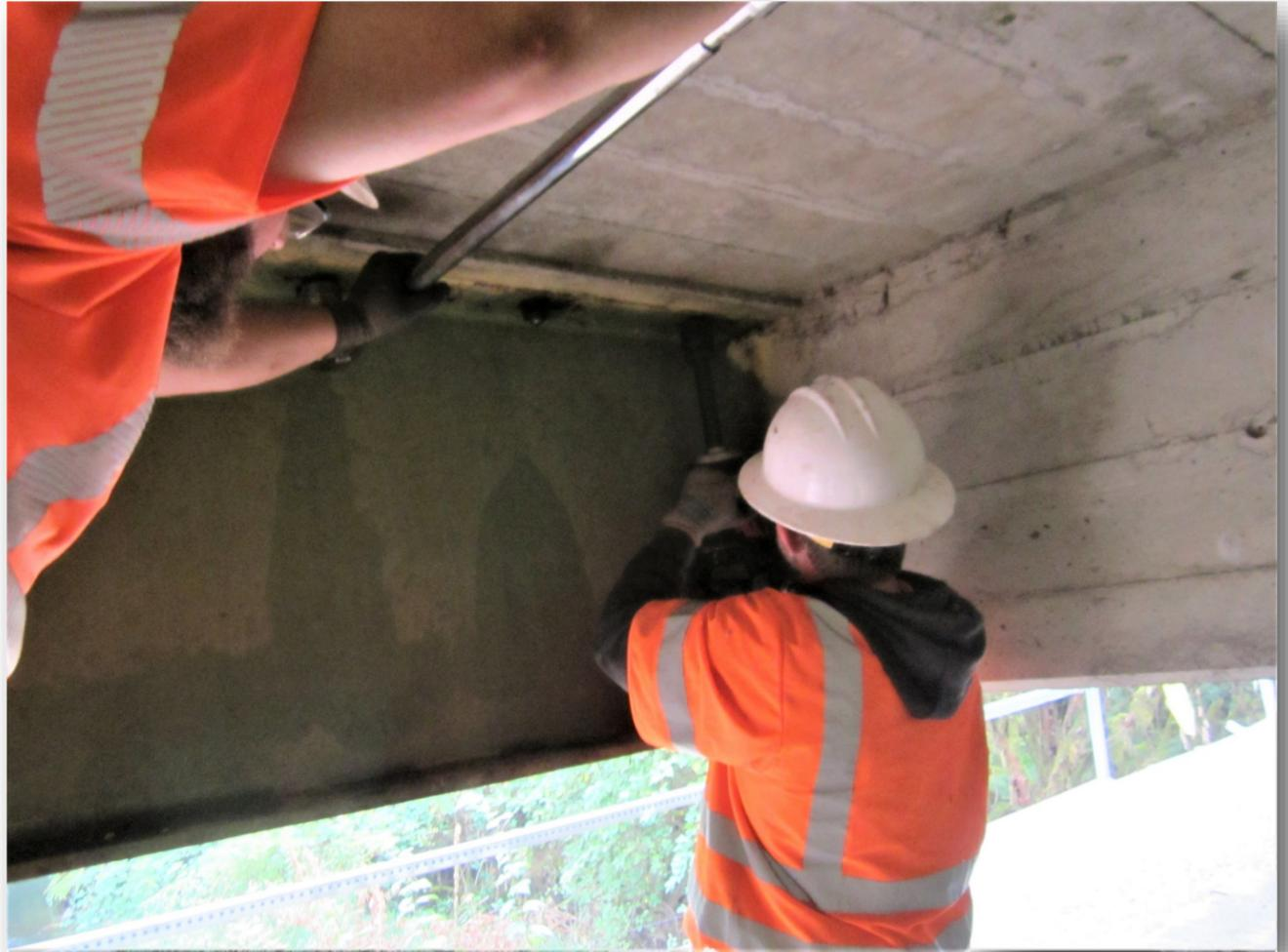
**Above:** Road Department staff install shear studs on a bridge on Lulay Road near Scio.
