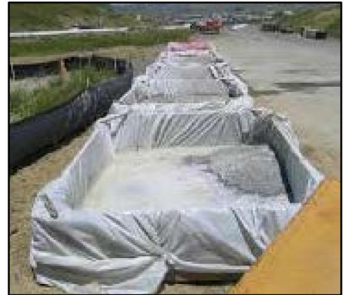
Image 3. Plastic Sheeting Lined Concrete Washout Basin
