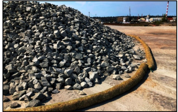
Image 1. Sediment Barrier at Parameter of Stockpile
