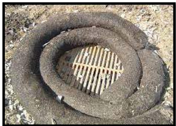
Image 2. Compost Filter Sock Inlet Protection
