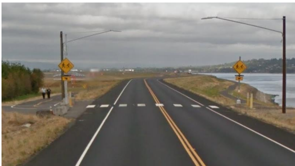
An example of an enhanced bicycle and pedestrian trail crossing with a Rectangular Rapid Flashing Beacon
